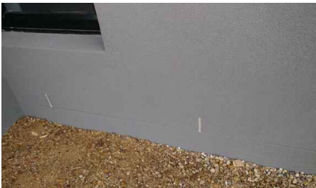
Weep holes/Vents: Found to be in serviceable condition when inspected
