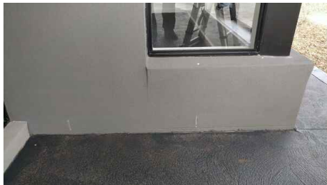
Weep holes/Vents: Found to be in serviceable condition when inspected
