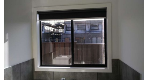
Window(s): In serviceable condition at time of inspection
